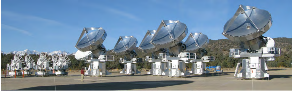
Figure 4.6: The Combined Array for Research in Millimeter-wave Astronomy (CARMA) is a university-based millimeter array consisting of six 10.4-meter, nine 6.1-meter, and eight 3.5-meter antennas that are used in combination at millimeter wavelengths. Located on a high-altitude site in eastern California, CARMA provides unparalleled sensitivity, broad frequency coverage, sub-arcsecond resolution and wide-field heterogeneous imaging capabilities, along with innovative technologies and educational opportunities. CARMA conducts cutting edge scientific research and provides unique learning opportunities for the next generation of instrumentalists and astronomers. CARMA is operated by the California Institute of Technology, University of California Berkeley, the University of Chicago, University of Illinois Champaign-Urbana, and the University of Maryland, with funding from the National Science Foundation and the member institutions.
